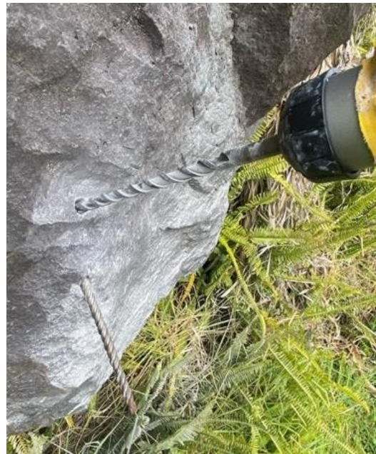
Using a spare drill bit as a guide to align the second hole. Photo: S. Fraser
